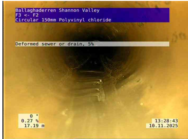
6, 00:02:35, 17.19 m Deformed sewer or drain, 5%
