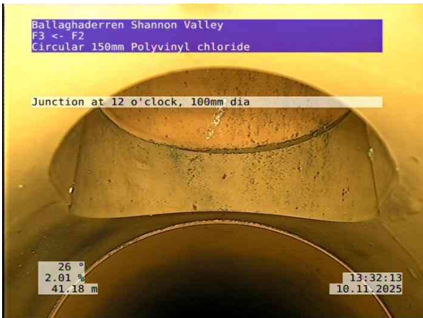
11, 00:05:42, 41.18 m Junction at 12 o'clock, 100mm dia
