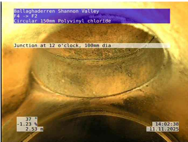
3, 00:00:40, 2.53 m Junction at 12 o'clock, 100mm dia
