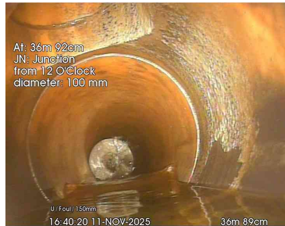
8, 00:03:05, 36.89 m Junction at 12 o'clock, 100mm dia
