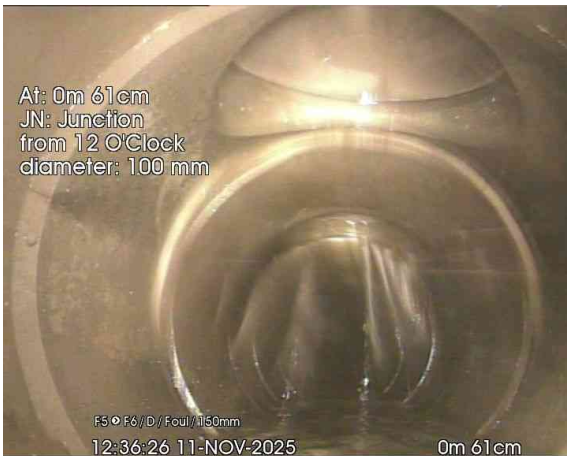
3, 00:00:15, 0.61 m Junction at 12 o'clock, 100mm dia
