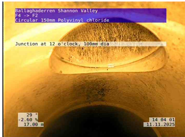
4, 00:02:01, 17.01 m Junction at 12 o'clock, 100mm dia
