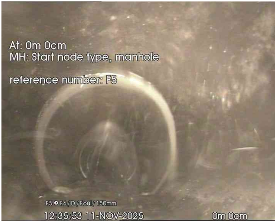
1, 00:00:01, 0.00 m Start node, manhole, reference: F5
