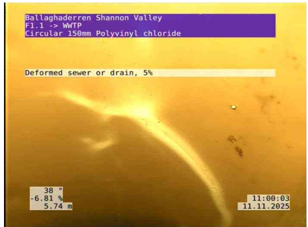
4, 00:01:09, 5.74 m Deformed sewer or drain, 5%
