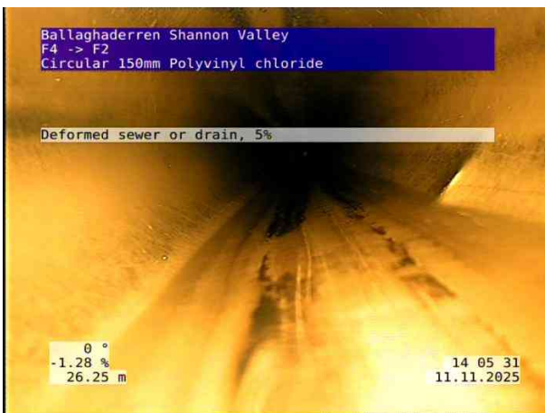
7, 00:03:14, 26.25 m Deformed sewer or drain, 5%
