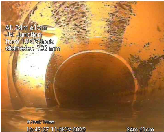
7, 00:01:32, 24.61 m Junction at 10 o'clock, 100mm dia
