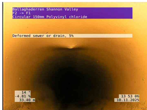
8, 00:04:48, 33.40 m Deformed sewer or drain, 5%
