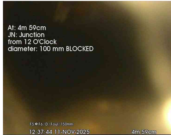
6, 00:00:55, 4.59 m Junction at 12 o'clock, 100mm dia, BLOCKED
