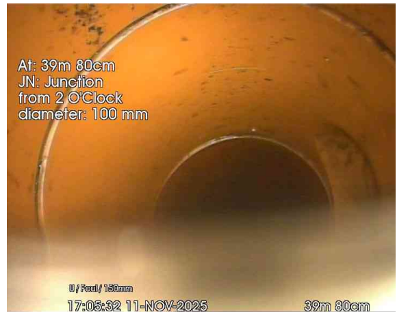
8, 00:04:29, 39.80 m Junction at 2 o'clock, 100mm dia
