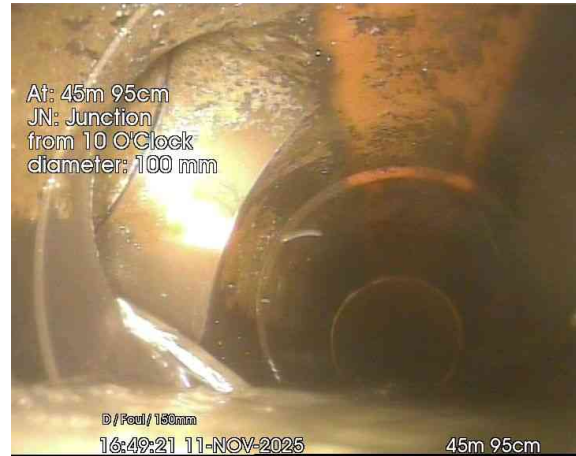
10, 00:02:48, 45.95 m Junction at 10 o'clock, 100mm dia
