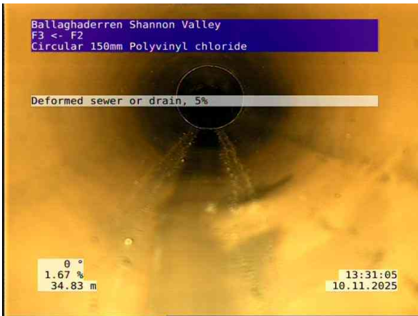
9, 00:04:44, 34.83 m Deformed sewer or drain, 5%
