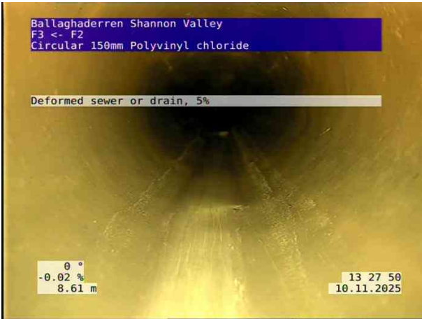
5, 00:01:45, 8.61 m Deformed sewer or drain, 5%
