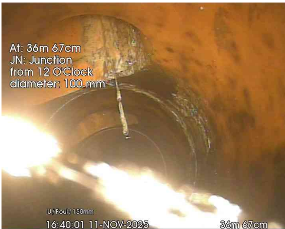
7, 00:02:57, 36.67 m Junction at 12 o'clock, 100mm dia
