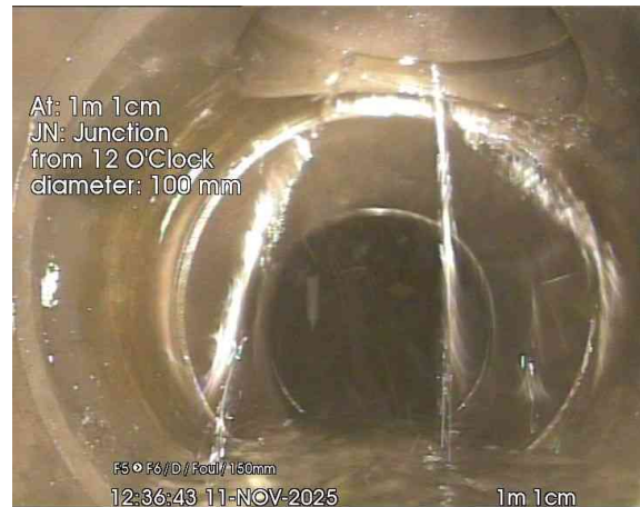
4, 00:00:23, 1.01 m Junction at 12 o'clock, 100mm dia
