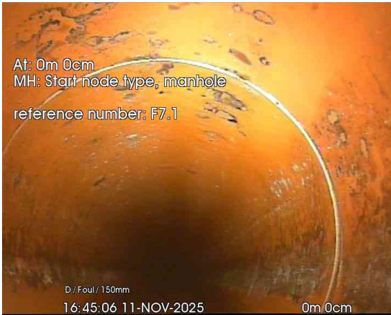
1, 00:00:01, 0.00 m Start node, manhole, reference: F7.1
