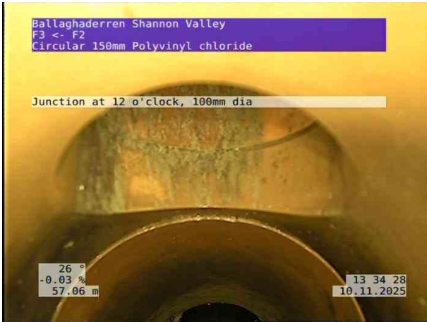
13, 00:07:48, 57.06 m Junction at 12 o'clock, 100mm dia
