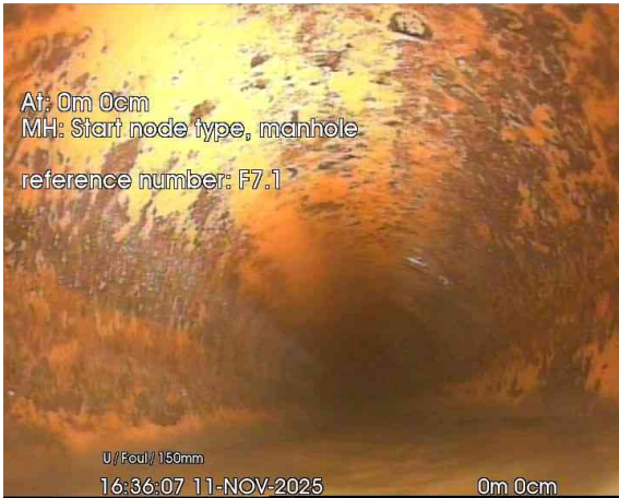
1, 00:00:01, 0.00 m Start node, manhole, reference: F7.1
