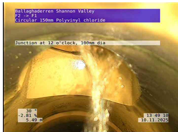
4, 00:01:12, 5.49 m Junction at 12 o'clock, 100mm dia
