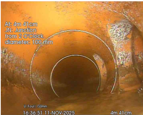
3, 00:00:26, 4.41 m Junction at 2 o'clock, 100mm dia
