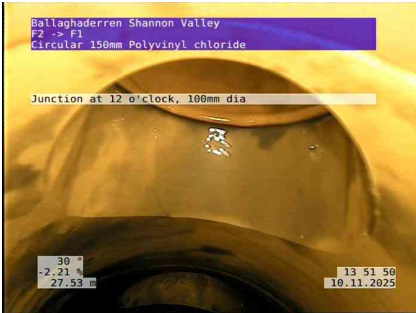
5, 00:03:44, 27.53 m Junction at 12 o'clock, 100mm dia
