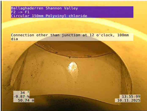
9, 00:06:42, 50.74 m Connection other than junction at 12 o'clock, 100mm dia
