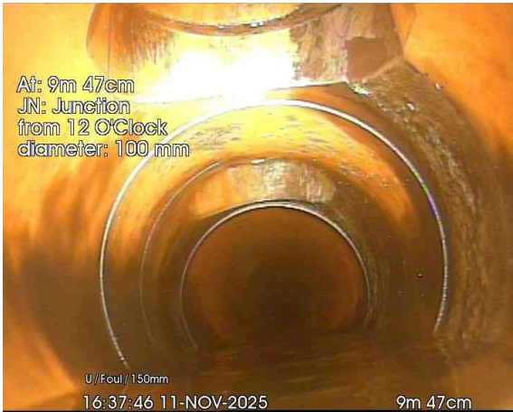
5, 00:01:02, 9.47 m Junction at 12 o'clock, 100mm dia
