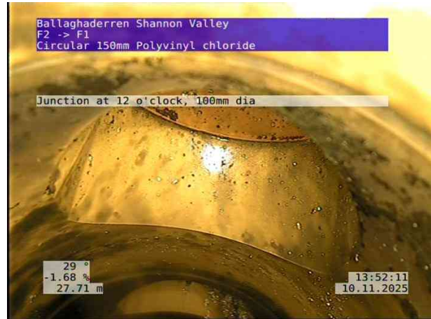
6, 00:04:01, 27.71 m Junction at 12 o'clock, 100mm dia
