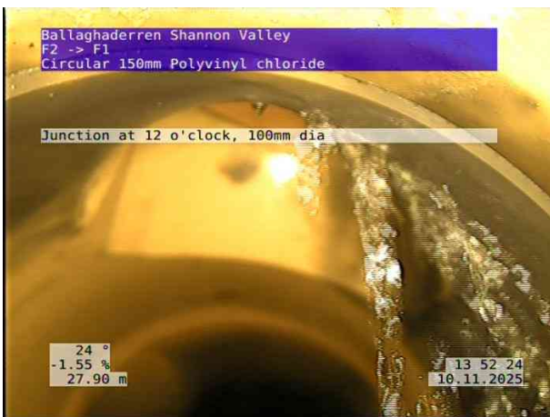
7, 00:04:10, 27.90 m Junction at 12 o'clock, 100mm dia
