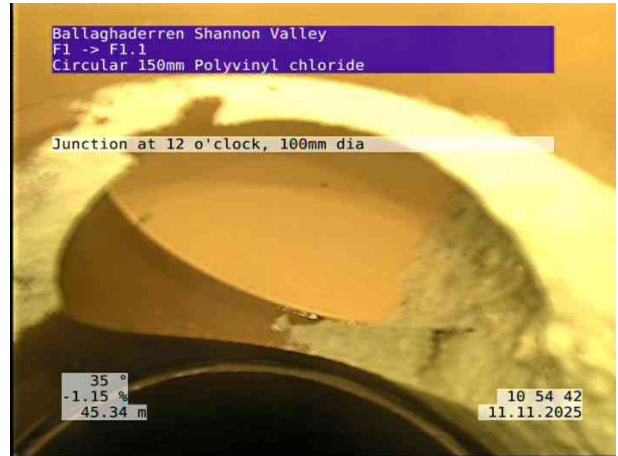
6, 00:05:06, 45.34 m Junction at 12 o'clock, 100mm dia
