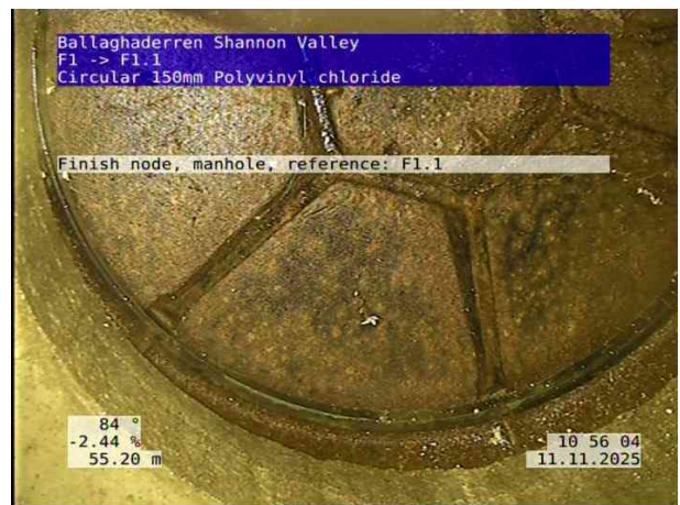
8, 00:06:09, 55.20 m Finish node, manhole, reference: F1.1
