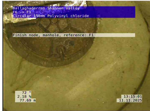
2, 00:07:07, 77.70 m Finish node, manhole, reference: F1
