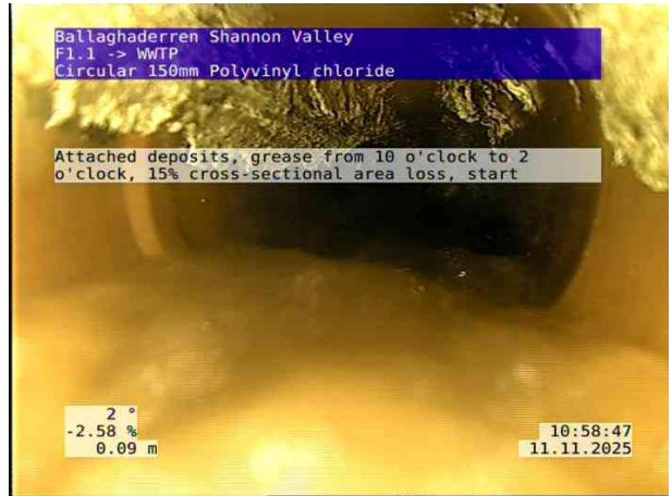
2, 00:00:10, 0.09 m Attached deposits, grease from 10 o'clock to 2 o'clock, 15% cross-sectional area loss, start
