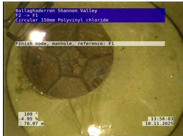
12, 00:09:15, 70.07 m Finish node, manhole, reference: F1
