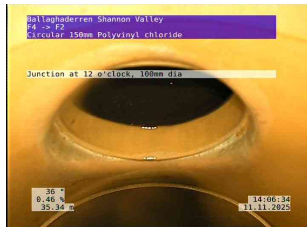
8, 00:04:11, 35.34 m Junction at 12 o'clock, 100mm dia
