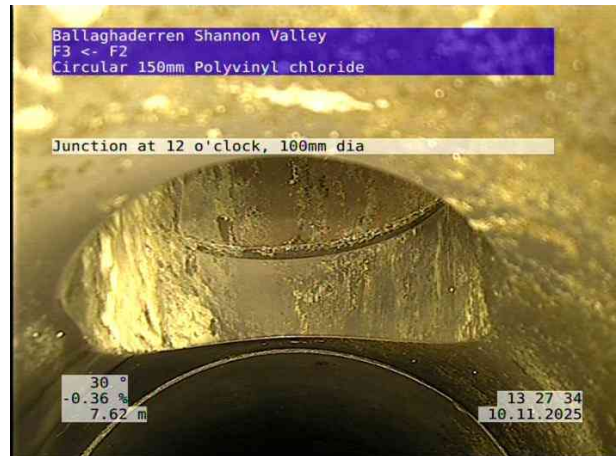
4, 00:01:33, 7.62 m Junction at 12 o'clock, 100mm dia
