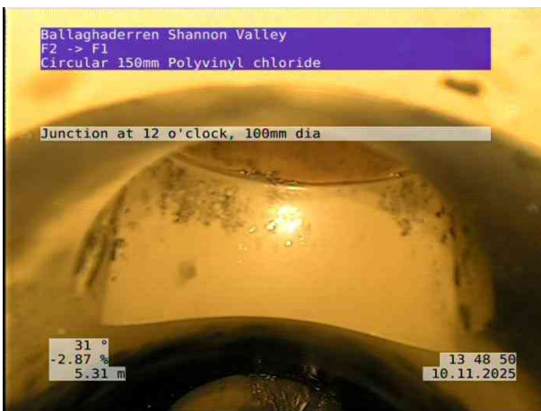
3, 00:00:58, 5.31 m Junction at 12 o'clock, 100mm dia
