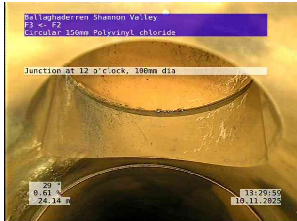
8, 00:03:41, 24.14 m Junction at 12 o'clock, 100mm dia
