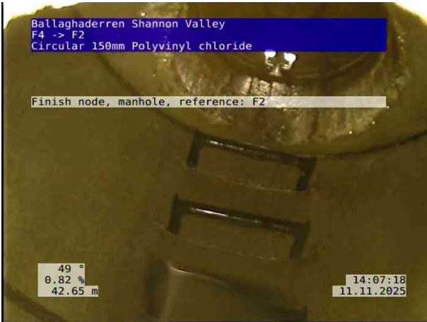
9, 00:04:51, 42.65 m Finish node, manhole, reference: F2
