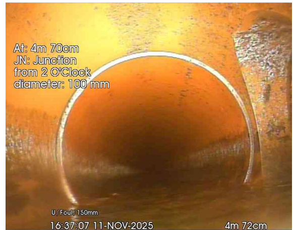
4, 00:00:33, 4.72 m Junction at 2 o'clock, 100mm dia
