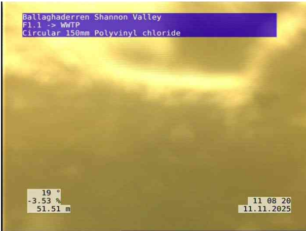
9, 00:07:01, 51.51 m Survey abandoned, CUW (HIGH WATER LEVEL AT PUMP STATION)
