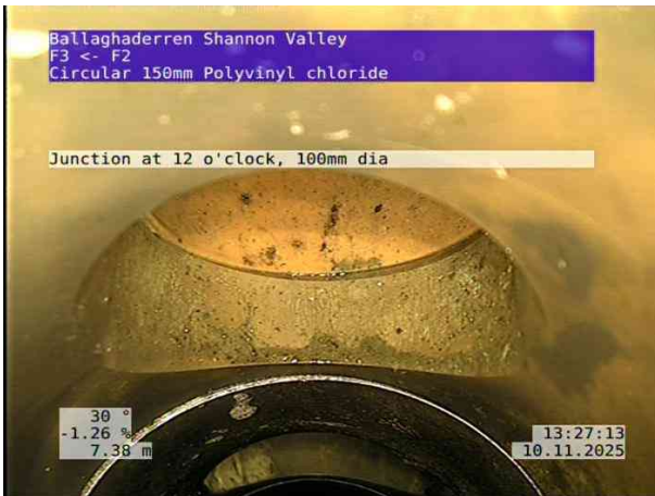
3, 00:01:17, 7.38 m Junction at 12 o'clock, 100mm dia
