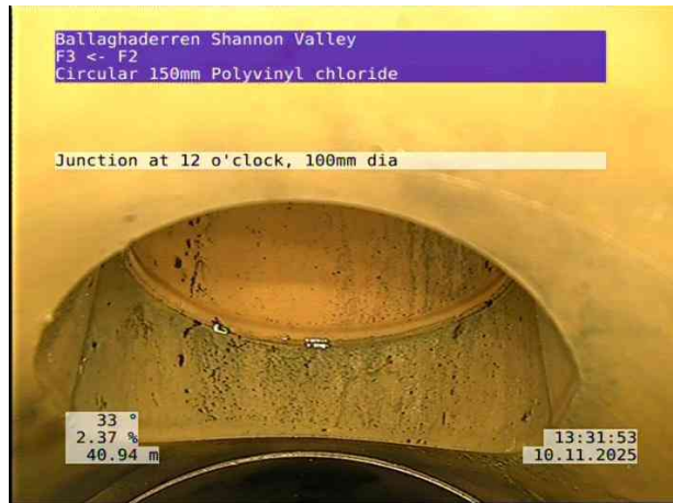
10, 00:05:27, 40.94 m Junction at 12 o'clock, 100mm dia
