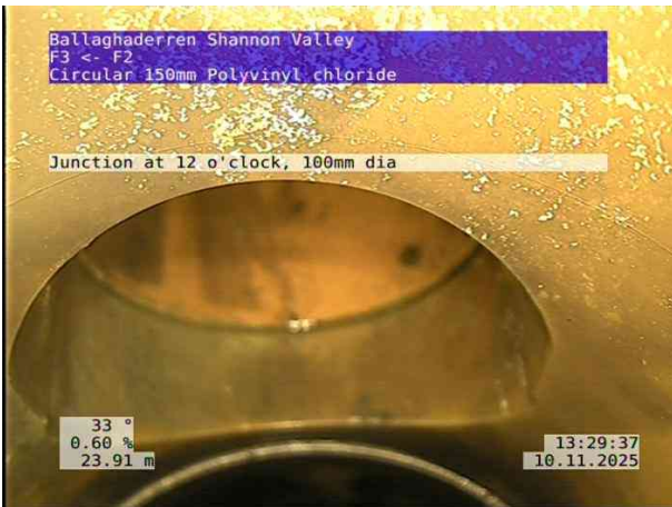
7, 00:03:24, 23.91 m Junction at 12 o'clock, 100mm dia
