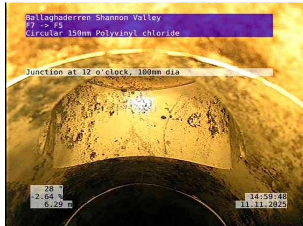
2, 00:01:23, 6.29 m Junction at 12 o'clock, 100mm dia
