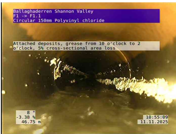
7, 00:05:21, 46.75 m Attached deposits, grease from 10 o'clock to 2 o'clock, 5% cross-sectional area loss
