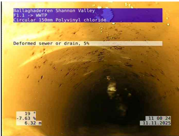
5, 00:01:28, 6.32 m Deformed sewer or drain, 5%
