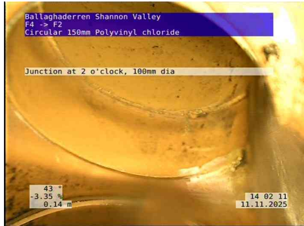
2, 00:00:18, 0.14 m Junction at 2 o'clock, 100mm dia
