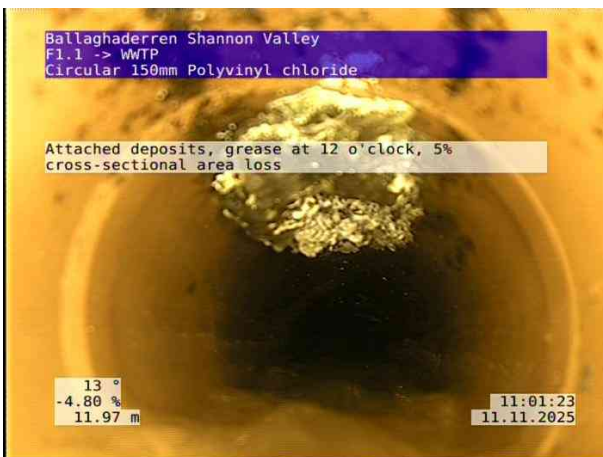
7, 00:02:08, 11.97 m Attached deposits, grease at 12 o'clock, 5% cross-sectional area loss
