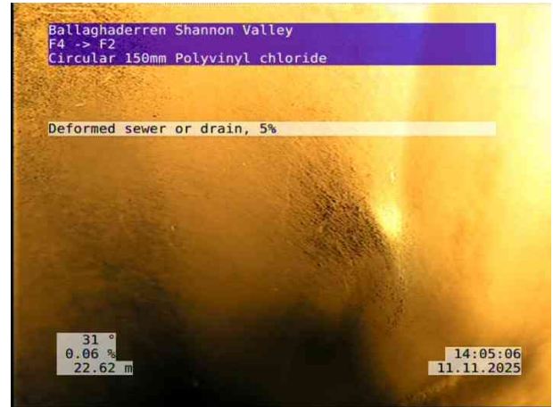
6, 00:02:53, 22.62 m Deformed sewer or drain, 5%
