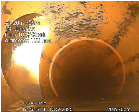
5, 00:01:14, 20.70 m Junction at 10 o'clock, 100mm dia
