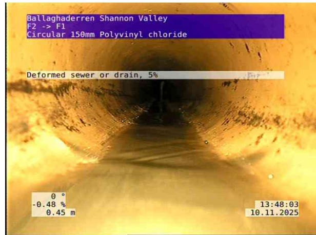
2, 00:00:16, 0.45 m Deformed sewer or drain, 5%
