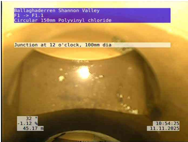
5, 00:04:53, 45.17 m Junction at 12 o'clock, 100mm dia
