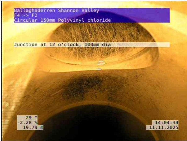
5, 00:02:29, 19.79 m Junction at 12 o'clock, 100mm dia
