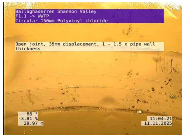
8, 00:03:58, 29.97 m Open joint, 35mm displacement, 1 - 1.5 x pipe wall thickness
