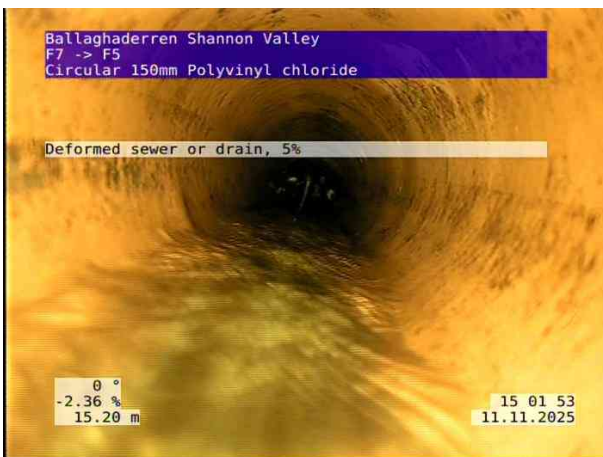
3, 00:03:09, 15.20 m Deformed sewer or drain, 5%
