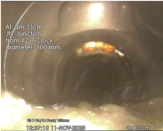
5, 00:00:49, 4.33 m Junction at 12 o'clock, 100mm dia
