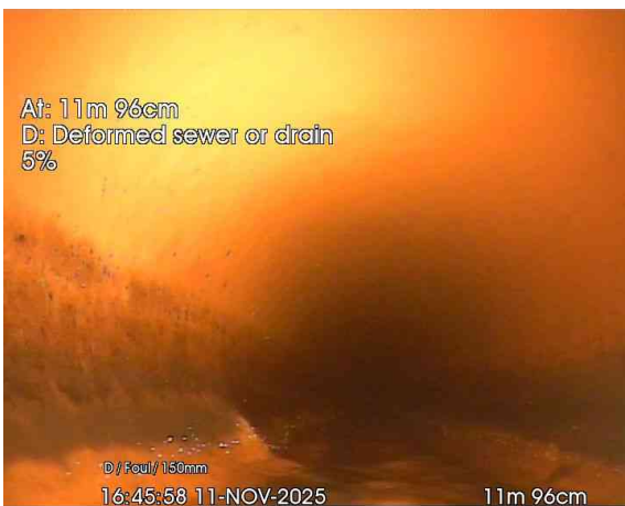
3, 00:00:38, 11.96 m Deformed sewer or drain, 5%
