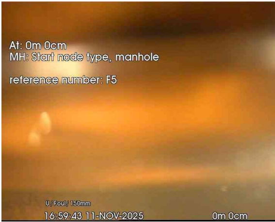
1, 00:00:01, 0.00 m Start node, manhole, reference: F5
