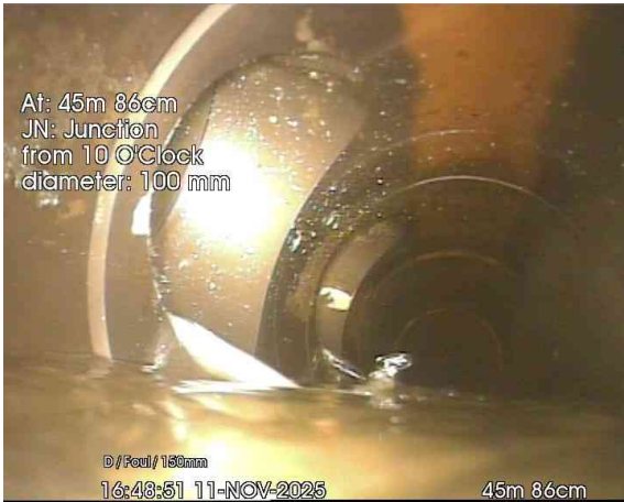
9, 00:02:37, 45.86 m Junction at 10 o'clock, 100mm dia
