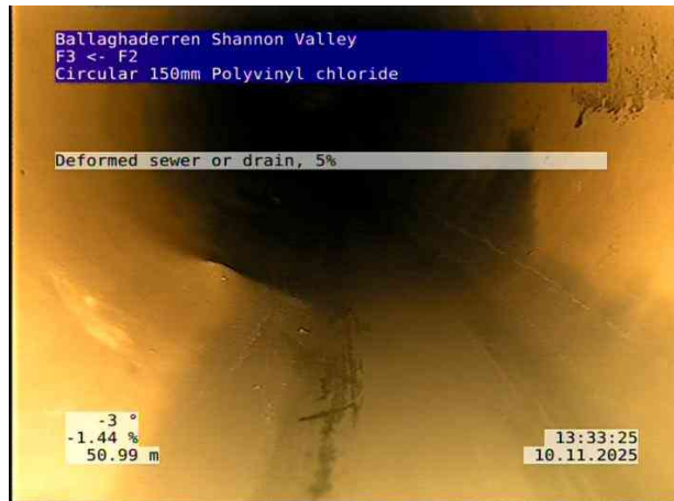
12, 00:06:52, 51.00 m Deformed sewer or drain, 5%
