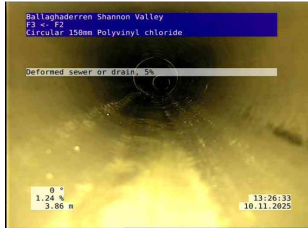
2, 00:00:41, 3.86 m Deformed sewer or drain, 5%
